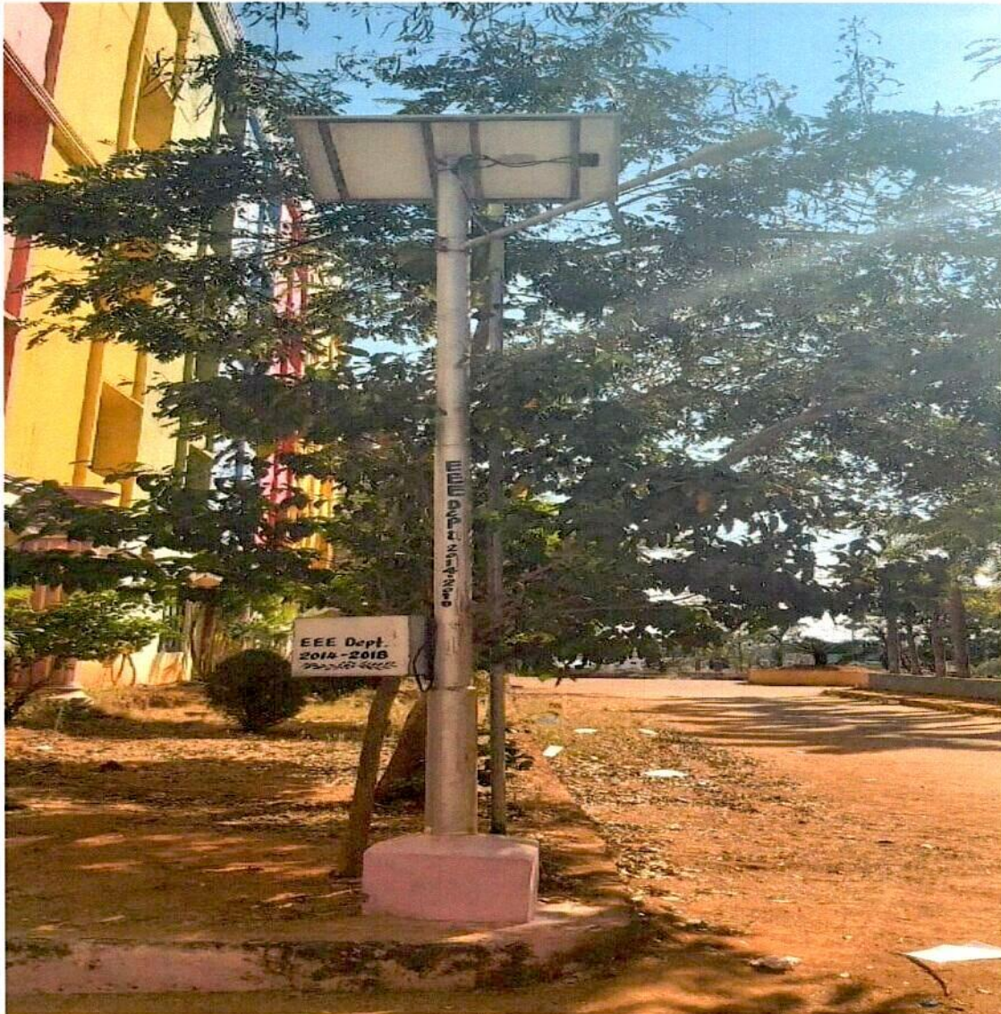
Sensor-Based solar power street lights in Campus.
